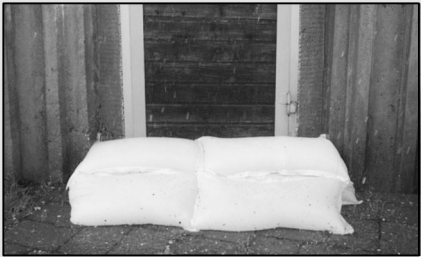
Protection of areas up to 100 cm wide e.g. doors, cellars, wells, ... We recommend to use 1-chamber sacks.
